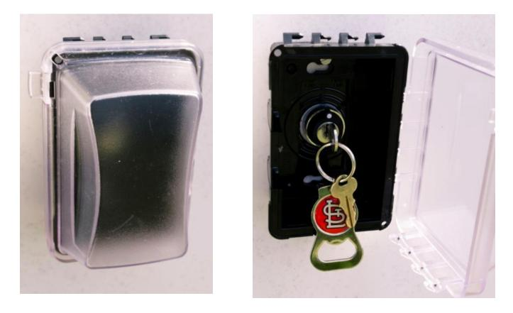
In order to open or close the shutter manually, I installed a key-operated momentary DPDT switch. This switch is wired in parallel with the manual switch mounted on the interface box. The key switch is mounted in a convenient location next to the shutter in a weather-proof box. The key is held in the appropriate position (open or close) until the shutter reaches the end of its travel and the limit switches remove power.
