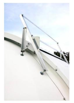
The 12VDC battery used to power the shutter windlass is kept charged by a solar panel (20 watt). Since my shutter faces north-south when closed I needed to devise a means of mounting the solar panel to face south at the appropriate angle. This was accomplished using aluminum channels attached to the dome by means of stainless steel eye-bolts. This arrangement allows the shutter to open and close sliding beneath the panel while providing a very light weight but sturdy mounting.
